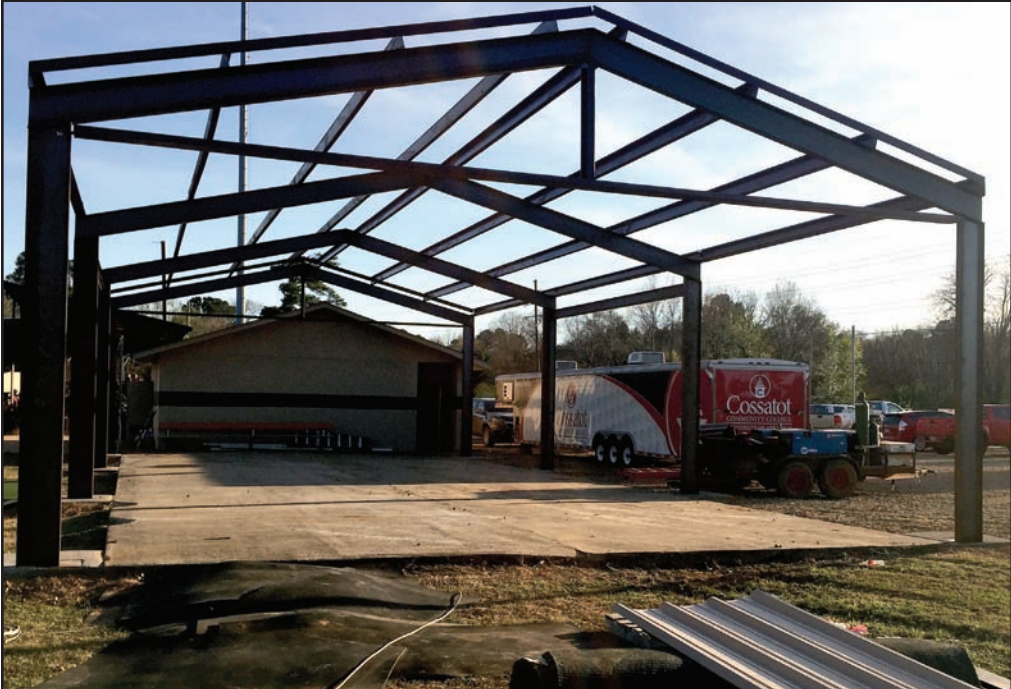
MORE WORK AT WILSON PARK. Construction of a batting cage is underway at the park. The project is sponsored by First State Bank and the school district.
