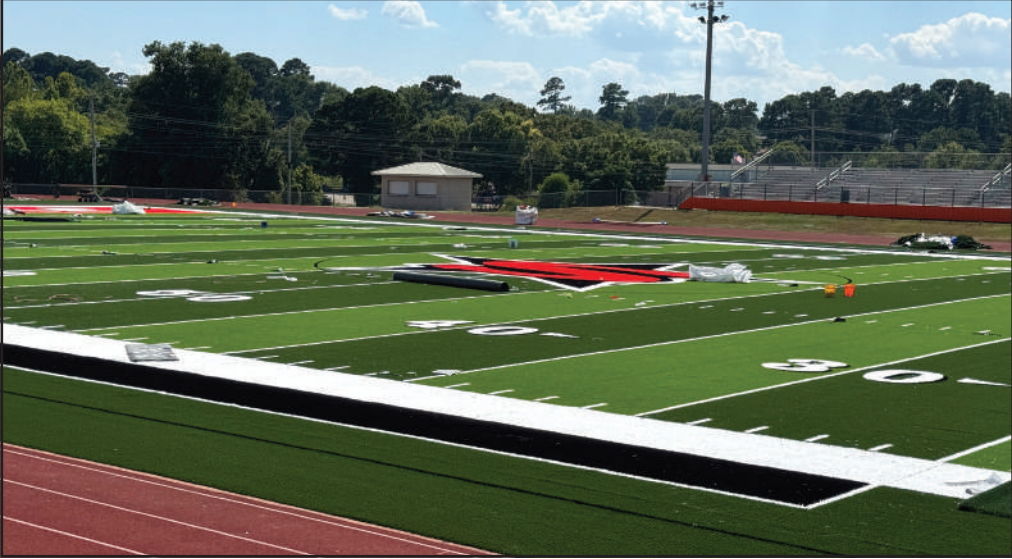
Work continues on the new artificial turf at Scrapper Stadium.
