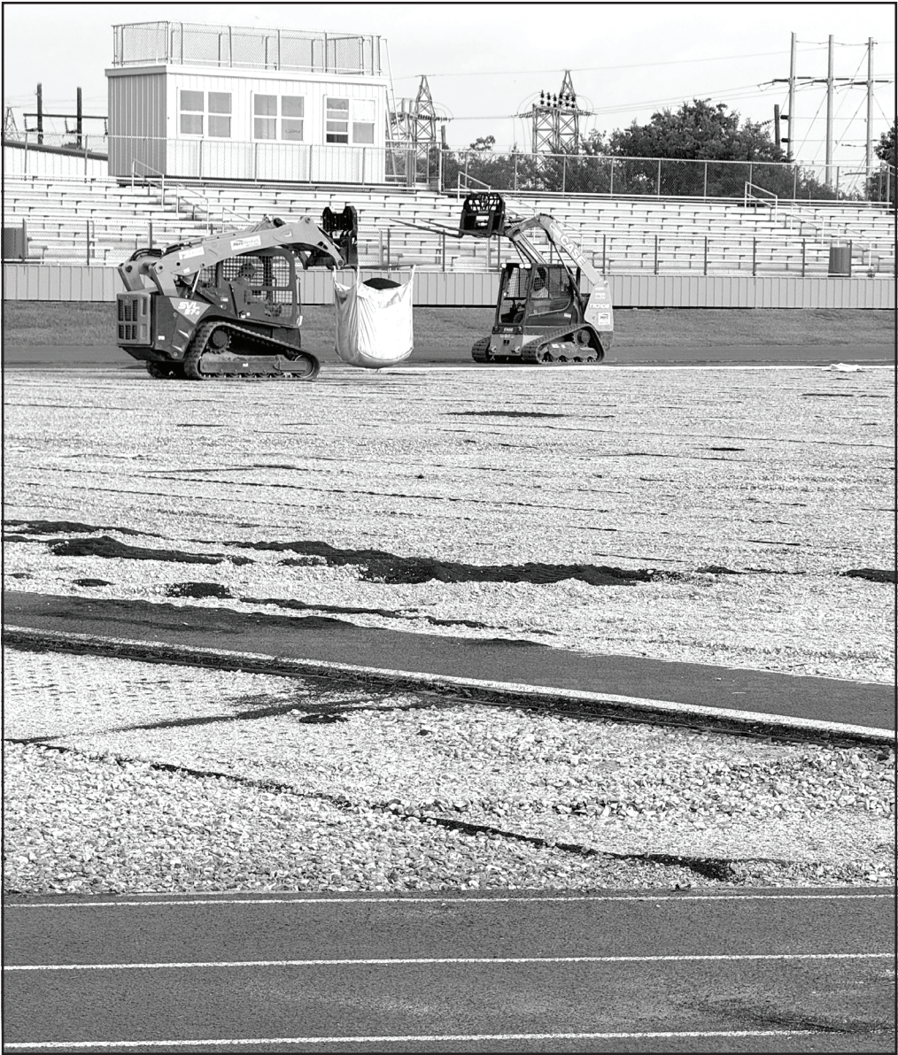
Crews haul off some of the debris after removing the stadium turf.
