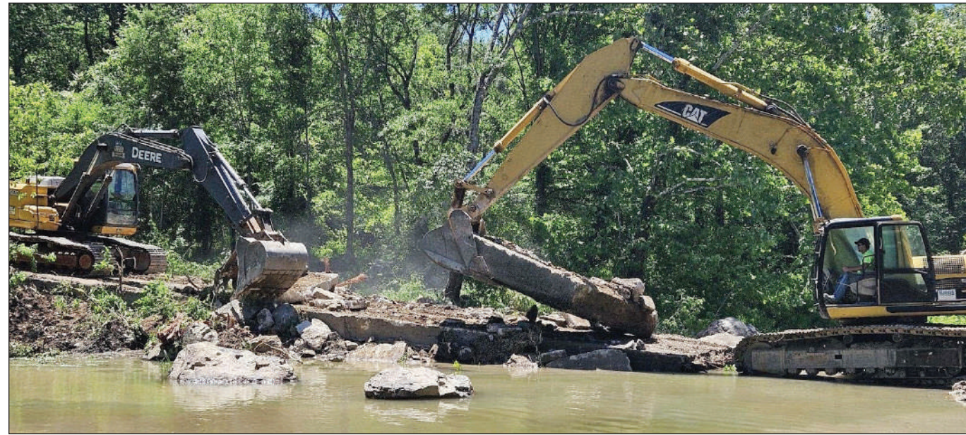
DEMO WORK. AGFC staff and contractors remove a low-water low-water crossing on the Rolling Fork River. AGFC photo.
