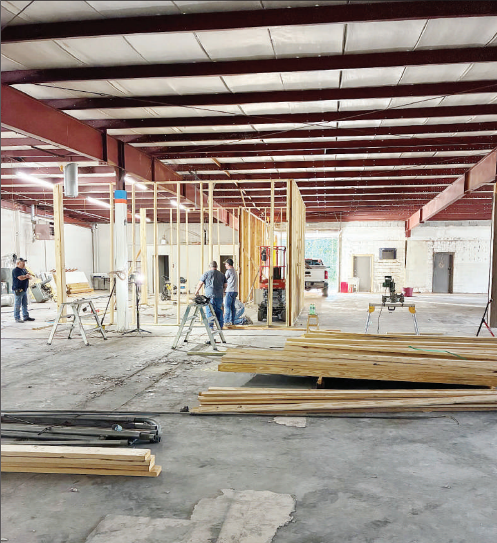
INSIDE WORK. The old Piggly Wiggly building’s transformation to a new grocery store for Murfreesboro is progressing for business owner Jack Bonds.
