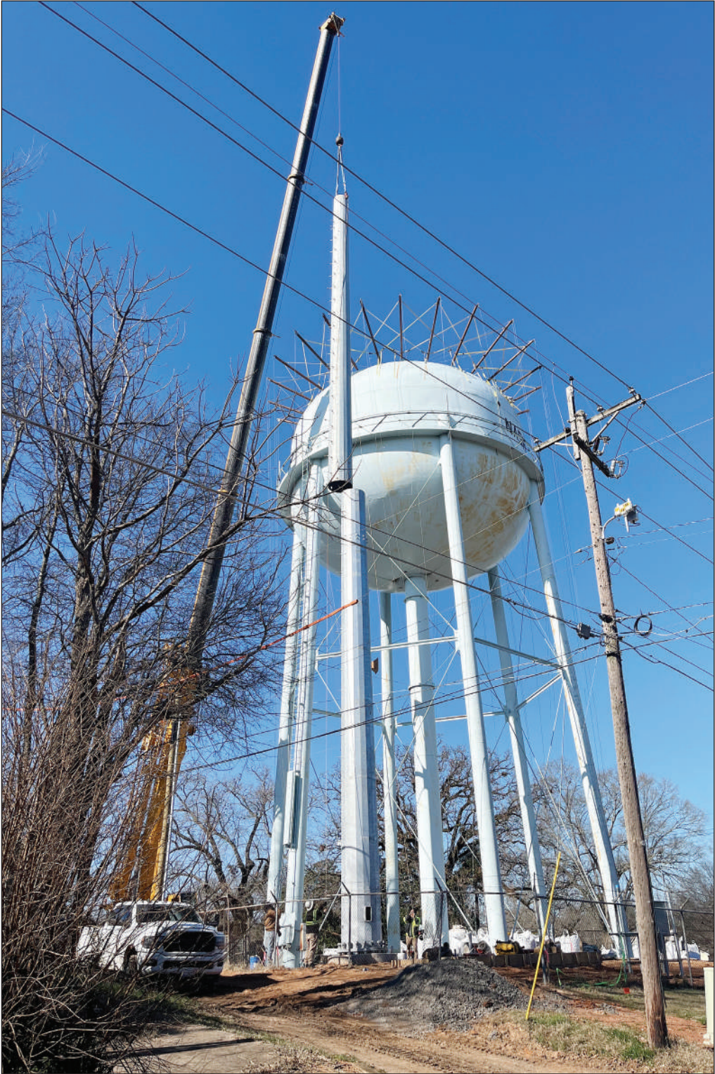
News-Leader photo/JOHN BALCH WORK CONTINUES ON TANK, CELL TOWER. Simultaneous work on Nashville's water tank on Third Street and the installation of an AT&T cell tower continues in the new year and should be completed by the end of the month, weather permitting. The tank is being sandblasted and painted and a big curtain will soon be up around the tower during the exterior painting. The tank has been isolated for the work and the water supply diverted to the tank on Seventh Street. Here, a large crane works beside the tank tower to install the second piece of the cell tower, which now stands several feet taller than the tank tower.
